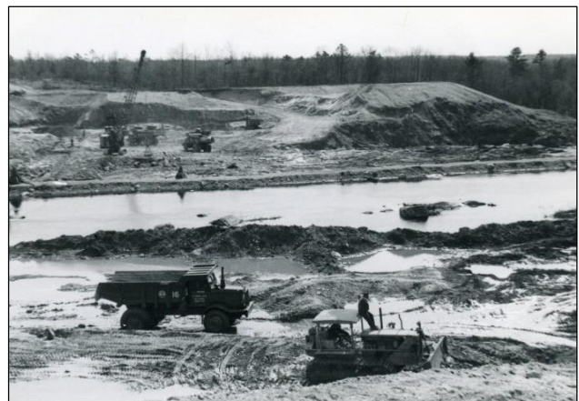
Constructing the Mansfield Hollow Dam, 1949-1952
